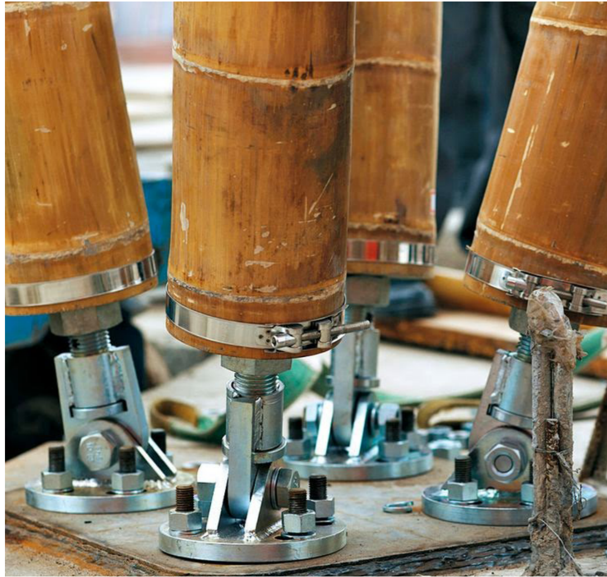
Reference image : Bamboo Pavilion pillar foundation pole architecture design
